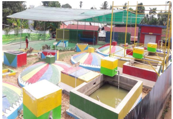
Figure 3 Biogas unit in Talang Banjar Jambi
