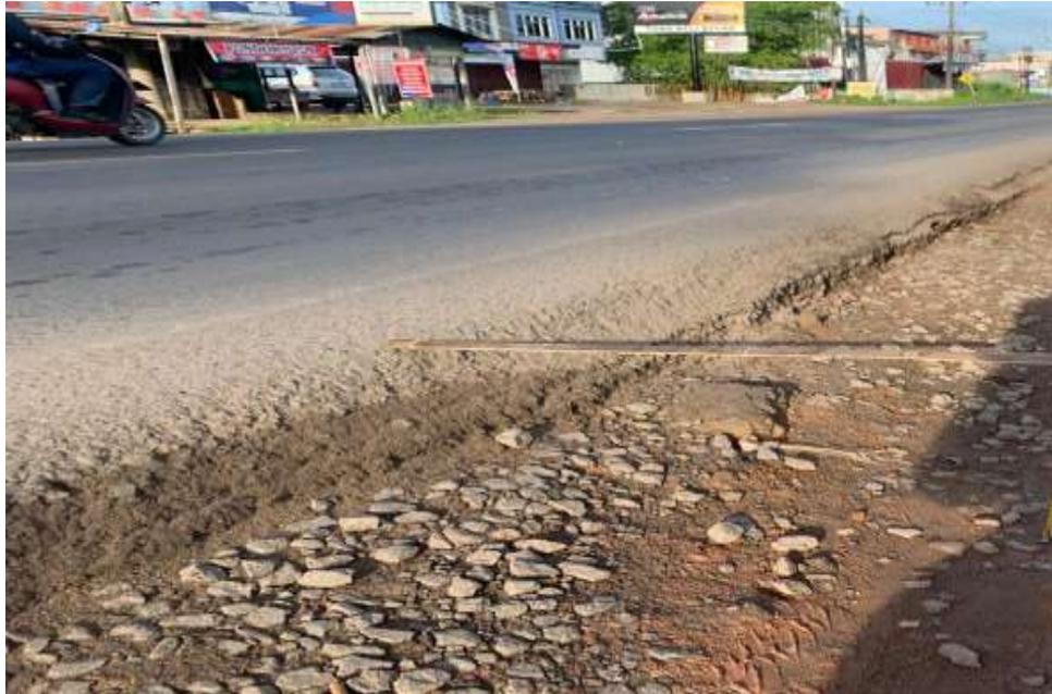
**Gambar 2.14** Penurunan Lajur/Bahu (*lane/shoulder drop off*)
