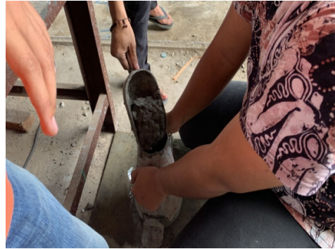
Proses pengujian slump test
