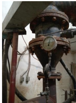
Gambar 2. 12 Outlet Check Valve
