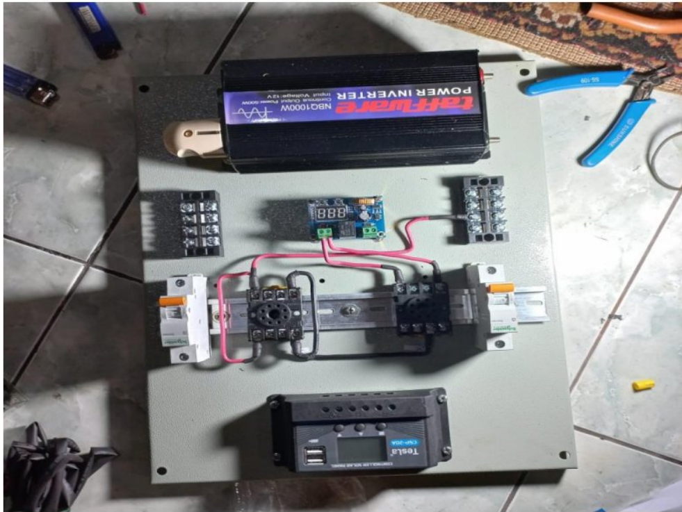
Proses perakitan panel box
