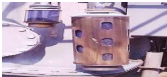
Gambar 2.7 Dehydrating Breather
