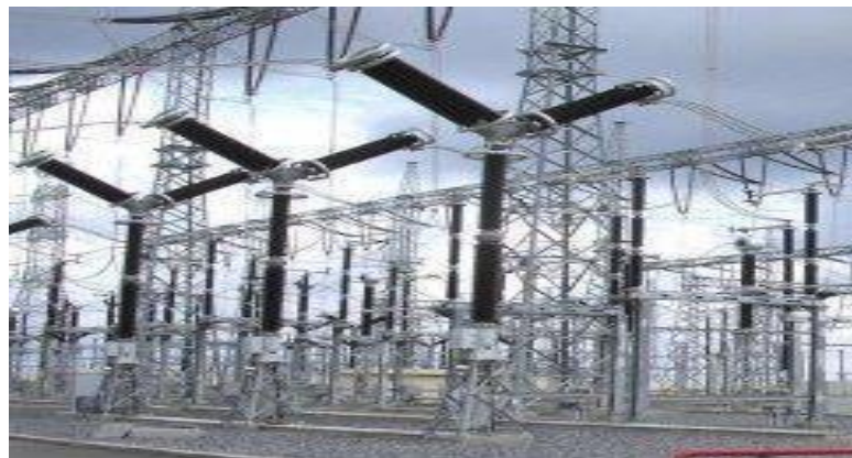
Gambar 2.6 PMT gas SF 6 [2]
