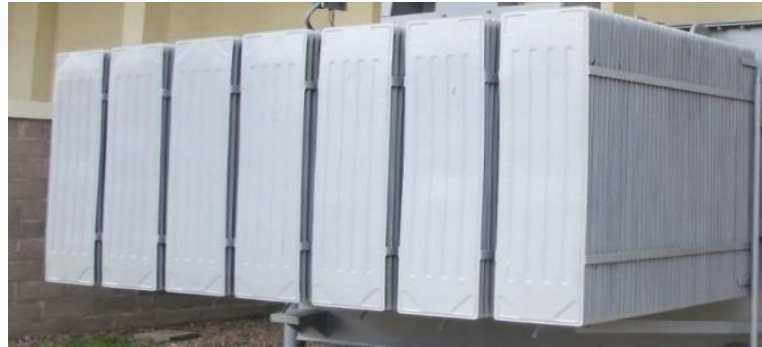
Gambar 2. 11 Pendingin Transformato
