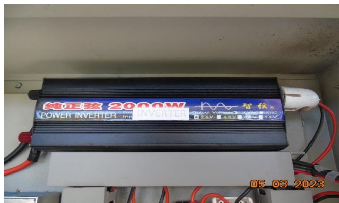
Gambar 2.3. Solar Power Inverter
