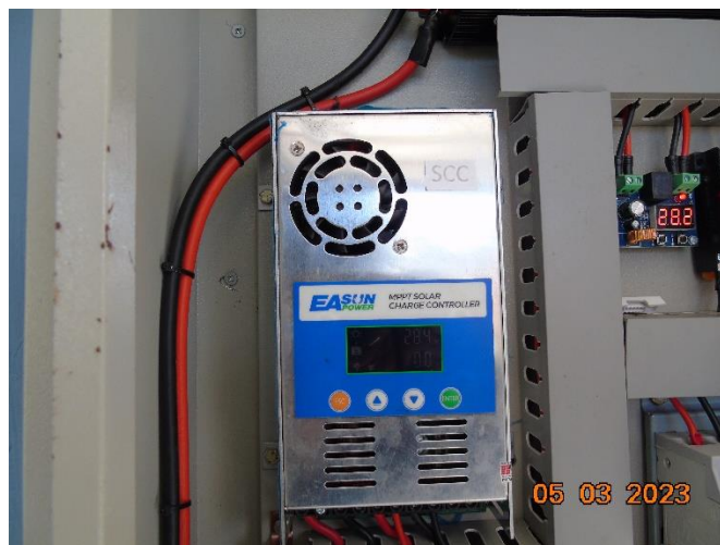
Gambar 2.2. Solar Charge Controller
