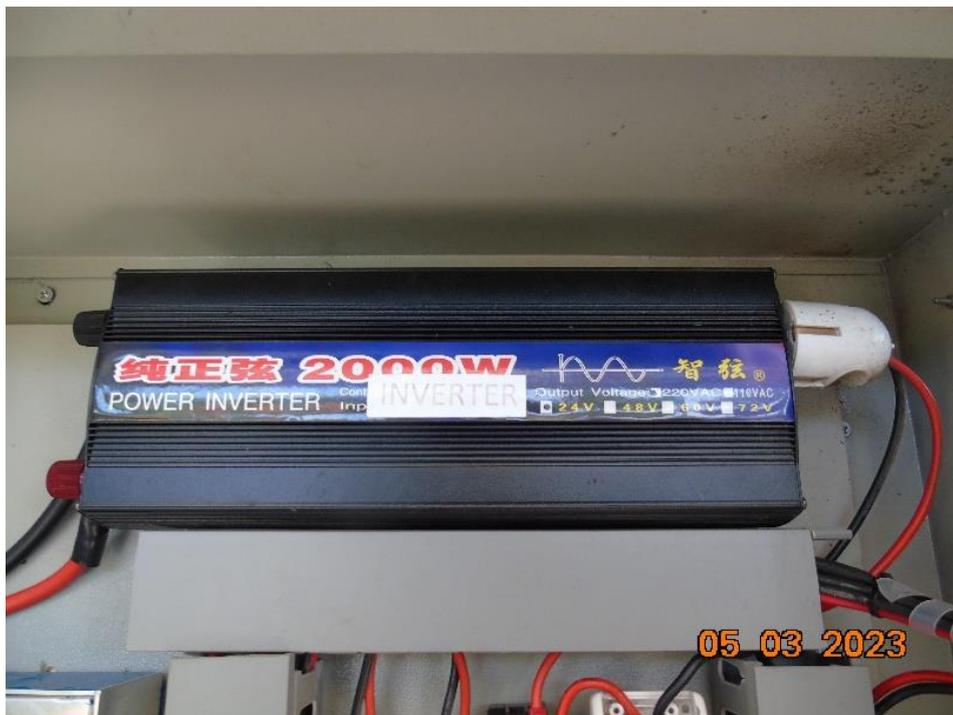
**Gambar 2.3.** *Solar Power Inverter*
