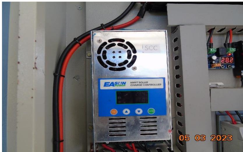
**Gambar 2.2.** *Solar Charge Controller*
