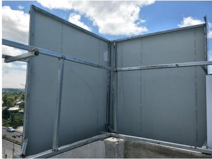
Gambar 2.18 Kerangka aluminium hollow + acp
