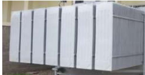
**Gambar 2.10 Pendingin Transformator**
