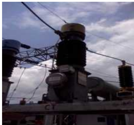
Gambar 2.3 Current Transformer
