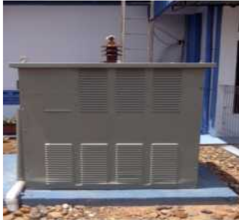
Gambar 2.2 Neutral Grounding Resistance
