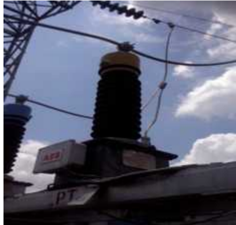
Gambar 2.4 Potential Transformer 3
