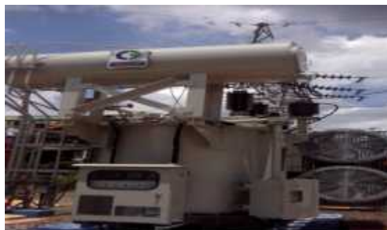
Gambar 2.1 Transformator Daya
