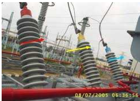
Gambar 2.13 Bushing Transformator
