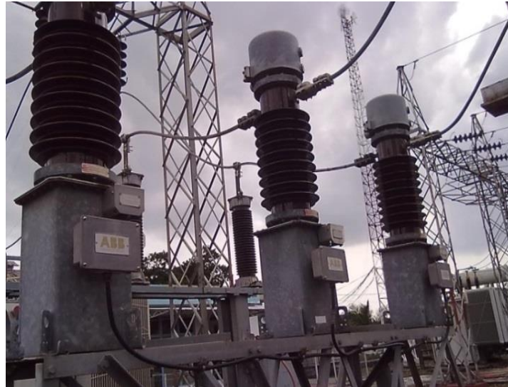
Gambar 2.20 Transformator Arus (CT) 25
