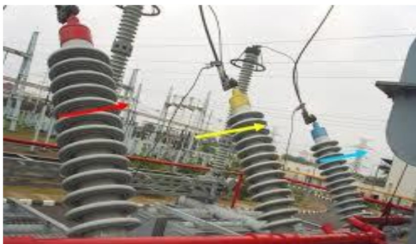
Gambar 2.4 Bushing Transformator
