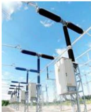
Gambar-2.10. SF<sub>6</sub> Gas Circuit Breaker
