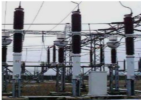
Gambar 2.6. Lightning arrester jenis gardu rating 150kV [6]
