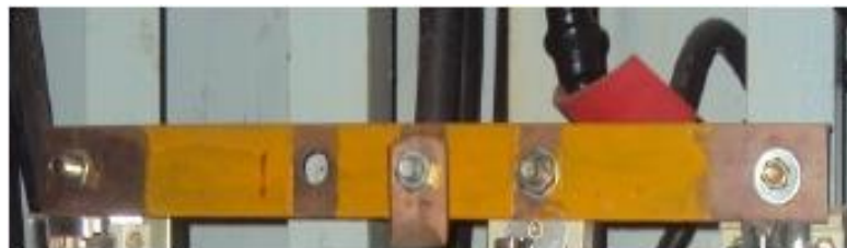
Gambar 2.5 Terminal Pbumian
