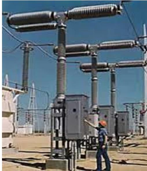
Gambar-2.12. SF6 Gas Circuit Breaker
