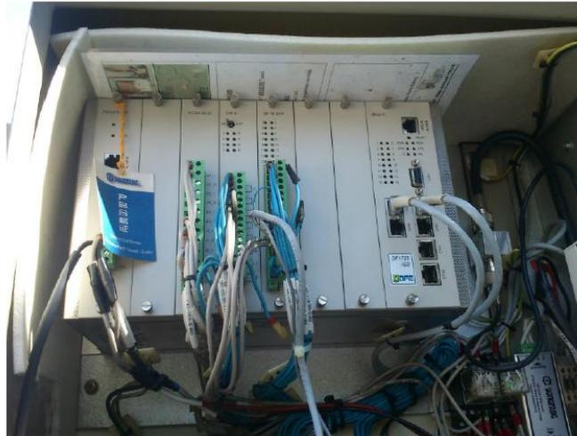
Gambar 2.13 Remote Terminal Unit (RTU)
