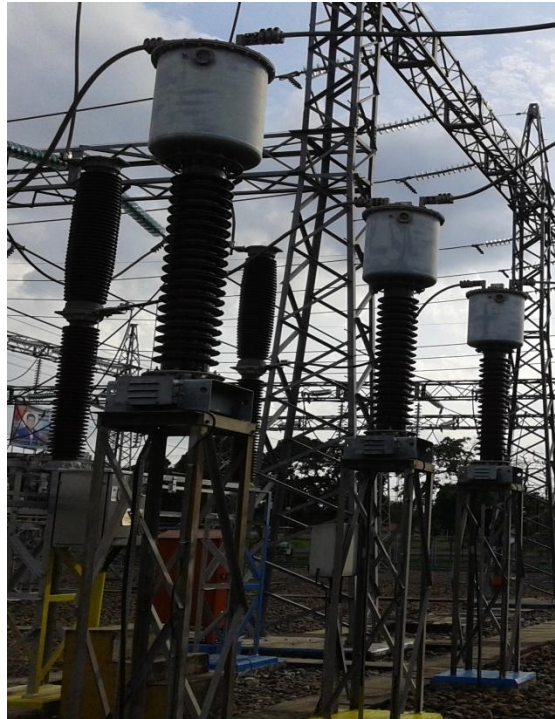
Gambar 3.3 CT Trafo 60 MVA II
