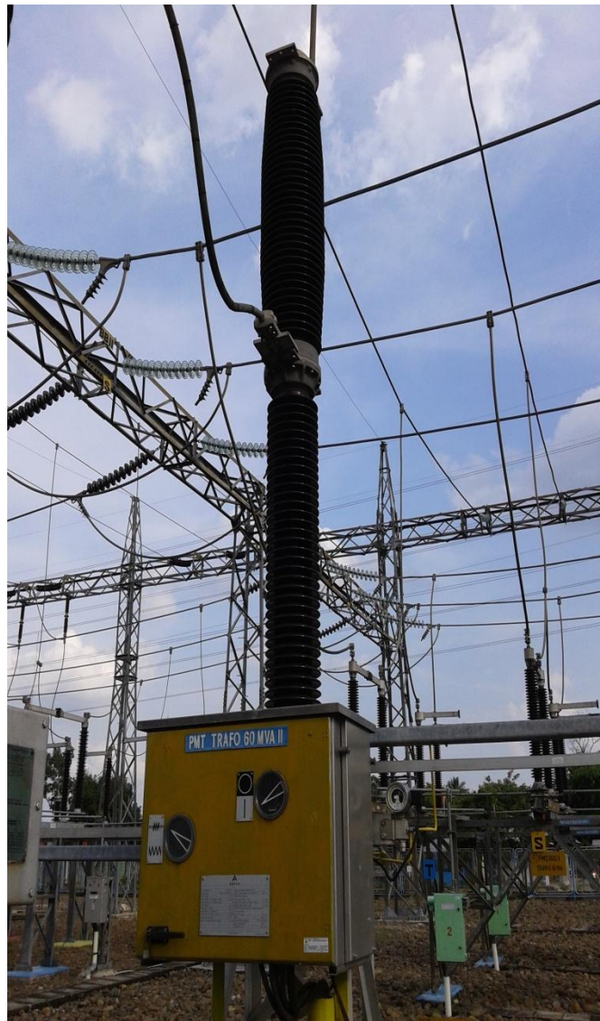
Gambar 3.2 PMT Trafo 60 MVA II
