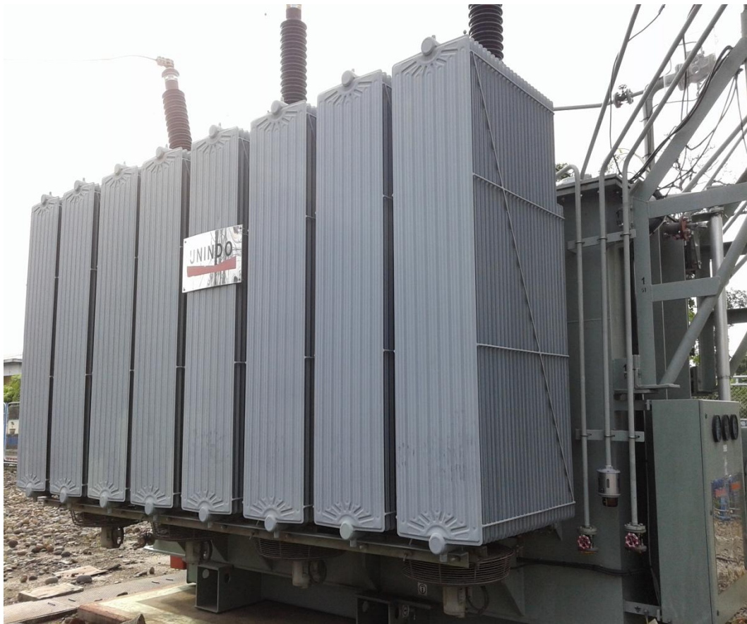
Gambar 3.1 Transformator Daya 60 MVA II
