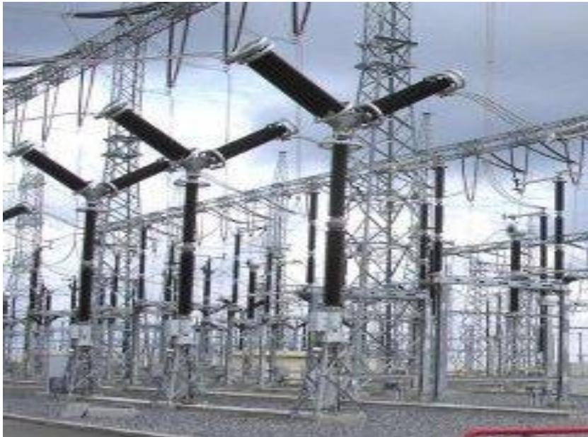
Gambar 2.8. SF<sub>6</sub> Circuit Breaker
