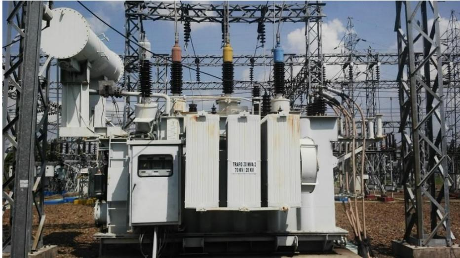
Gambar 2.12 Transformator Daya
