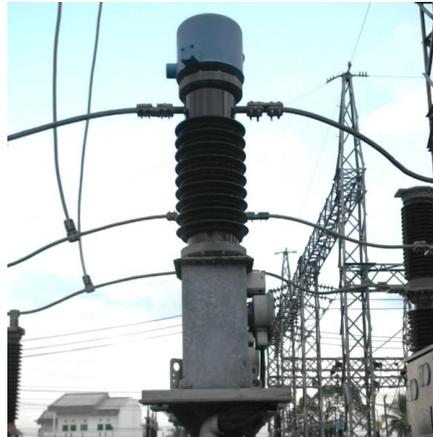
Gambar 2.20 Transformator Arus
