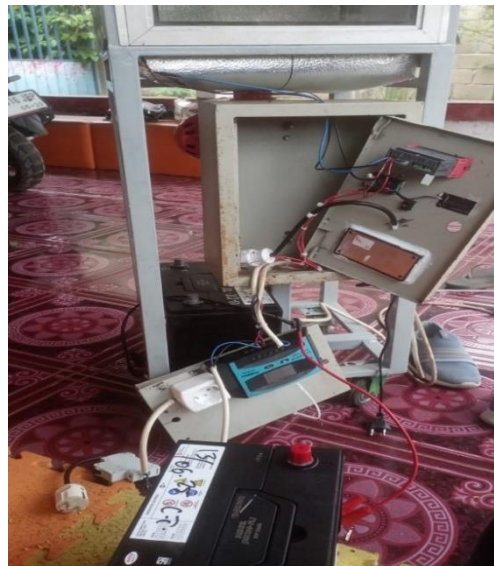
Gambar L3. 7 Merangkai Kabel Box Controller Panel Surya
