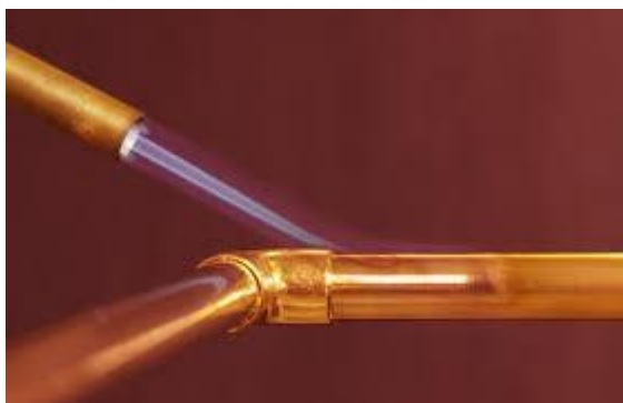
Gambar 2.6 Proses Soldering
