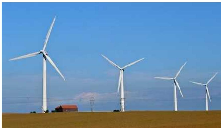
Gambar 2.1 Turbin Angin Sumbu Horizontal
