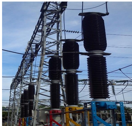
Gambar 2.10 SF 6 Circuit Breaker
