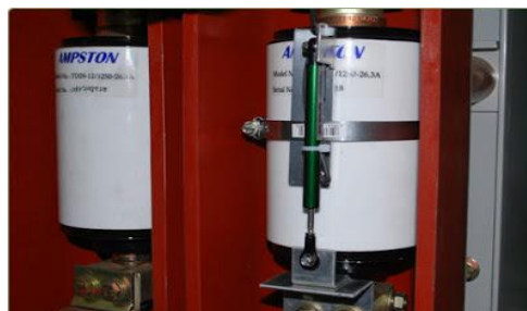
Gambar 2.9 Vacuum circuit breaker
