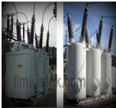
Gambar 2.6 Oil Circuit Breaker
