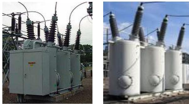
Gambar 2.8. PMT Bulk *oil*
