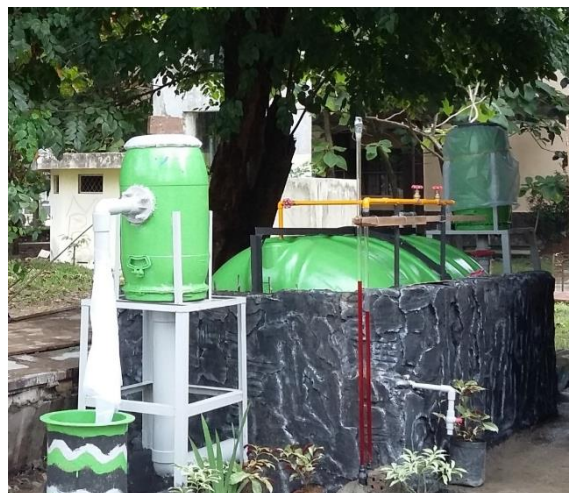
Fixed Dome Digester
