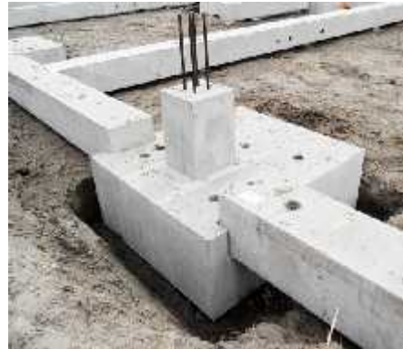
Fig. 2 Precast foundations
