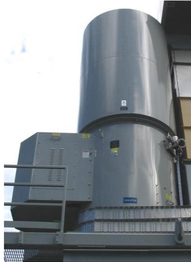
**Gambar 2.12 Turbine Enclosure Fan**
