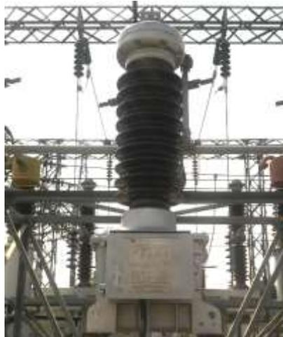
Gambar 2.17 Transformator Tegangan
