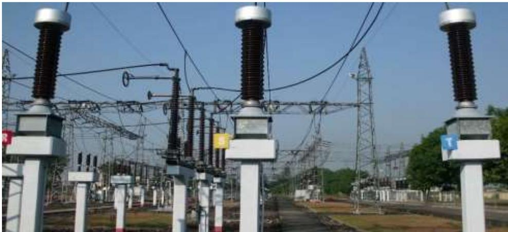
Gambar 2.16 Transformator Arus
