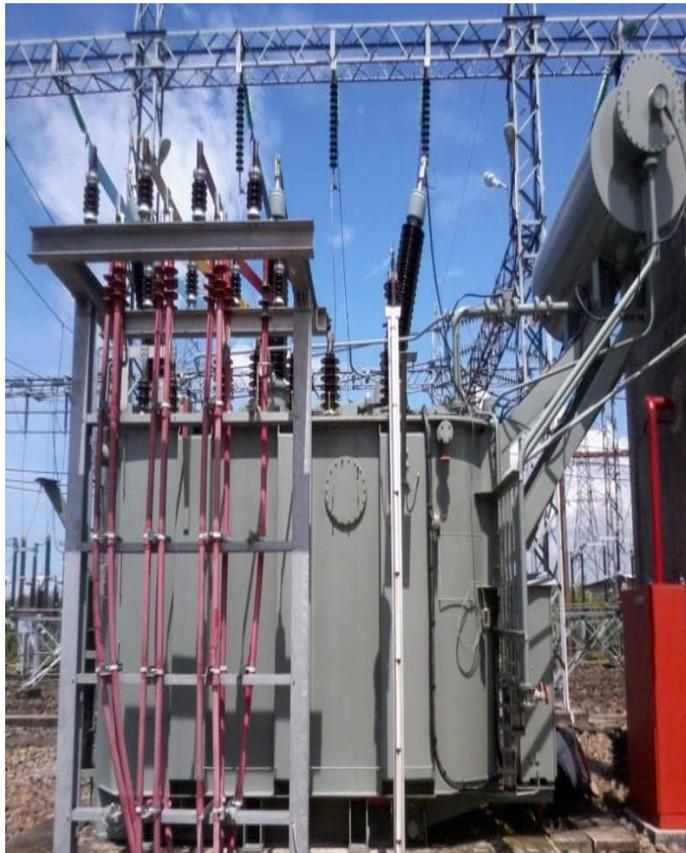
Gambar 2.1 Transformator daya
