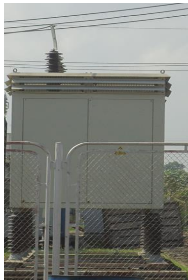
Gambar 2.17. Neutral grounding resistance (NGR)
