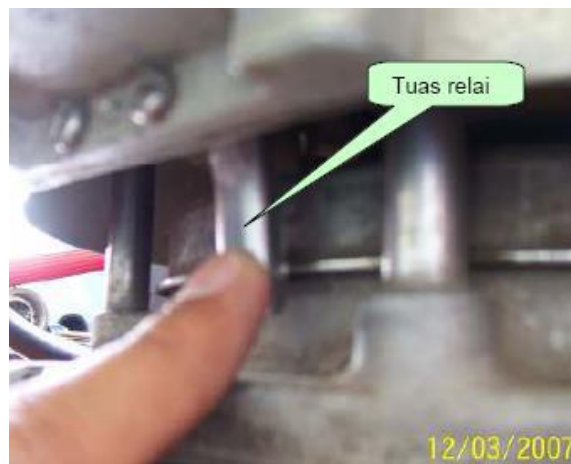
Gambar 2.50 tuas rele sudden pressure
