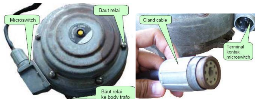
Gambar 2.36 rele sudden pressure
