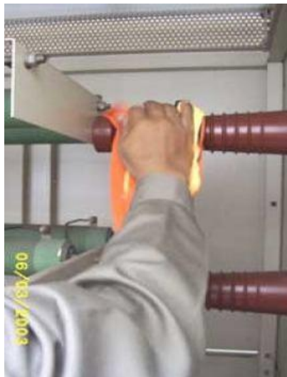
Gambar 2.51 Proses pembersihan ( Cleaning ) NGR
