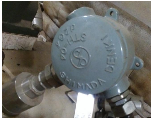
Gambar 2.11 Rele Over Speed
