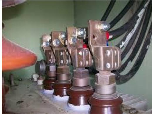
Gambar 2.4 Bushing Transformator
