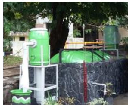
Gambar 25. Digester Fixed Dome Type
