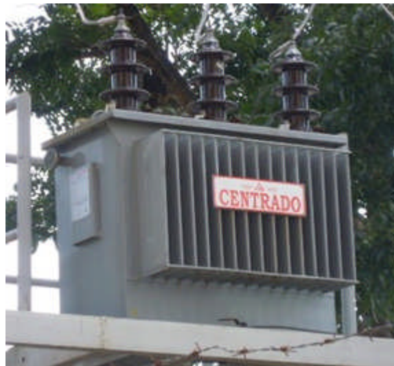
Gambar 2.1 Transformator 3 Phasa 2
