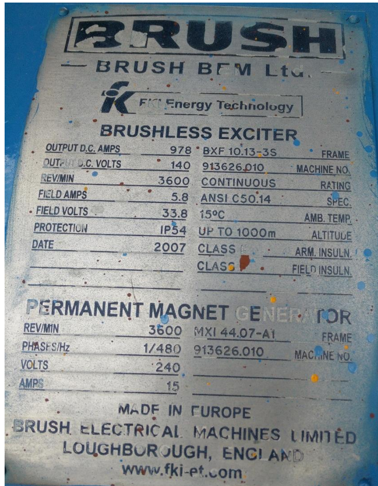
Gambar Namplate Exiter Generator Gas Unit TM2500 Unit #1 PLTG CNG Jakabaring
