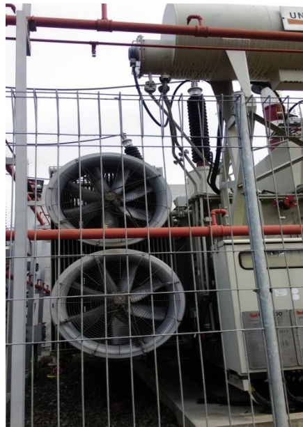
Gambar 2.10 Pendingin Transformator
