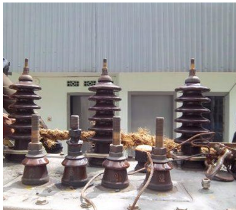
Gambar 2.8 Bushing Transformator
