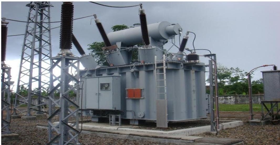
**Gambar 2.2** Transformator Daya
