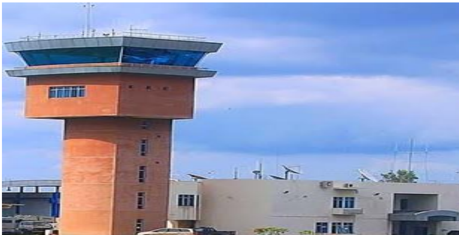
Gambar 2.10 Air Traffic Control Tower
