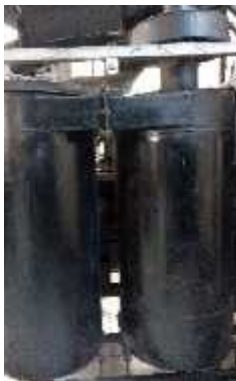
Gas Cooler dan Filter
