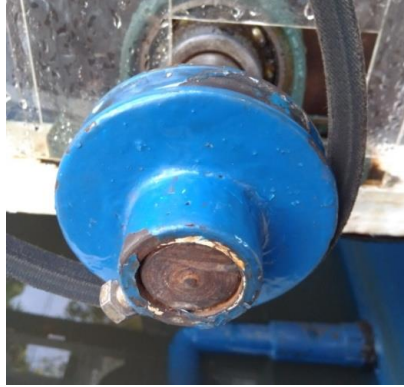
Gambar L2.4 Pulley Turbin Air
