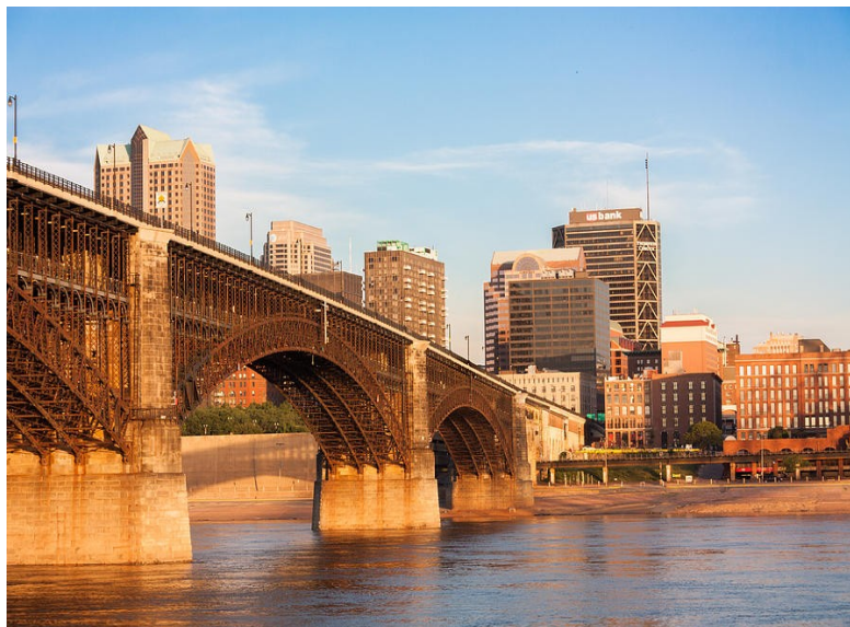
Gambar 2.4 Eads Bridge, St. Louis, USA ( Sumber : www.bridgepos.com )
