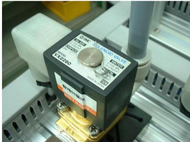
**Gambar 2.10** Solenoid valve 12V DC
