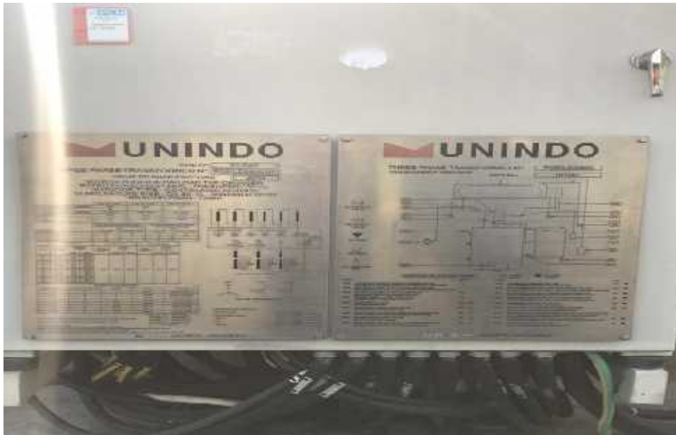
Gambar 3.2 Name plate transformator daya 54 MVA
