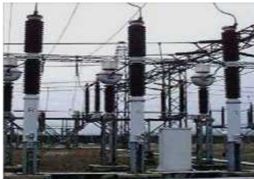
Gambar 2.6. Lightning arrester jenis gardu rating 150kV [6]
