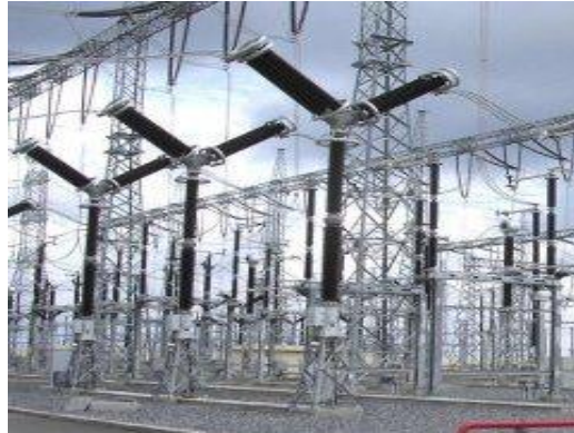
Gambar 2.9. SF 6 Circuit Breaker 11
