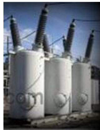
Gambar 2.4. Oil Circuit Breaker 5
