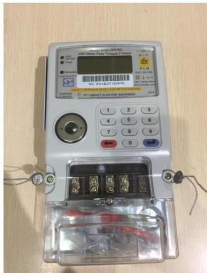
Gambar 2.6 Kwh meter digital
