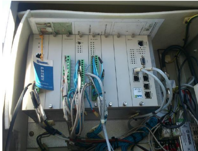
Gambar 2.17 Remote Terminal Unit (RTU)
