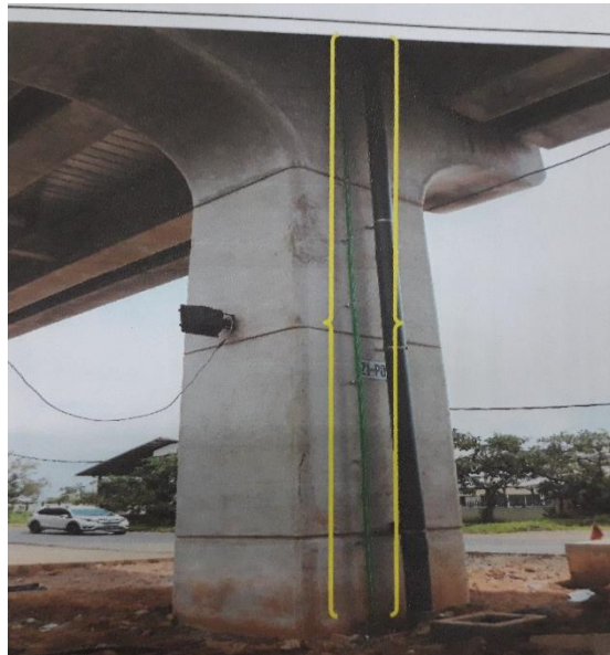
Gambar 2.12 Master Grounding Line
