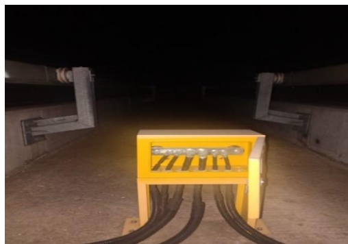
Gambar 2.11 Box terminal SCC
