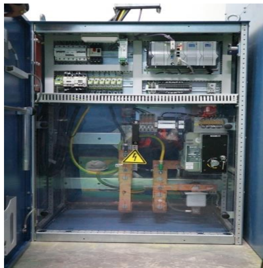
Gambar 2.18 Voltage Limiting Device Tampak Depan
