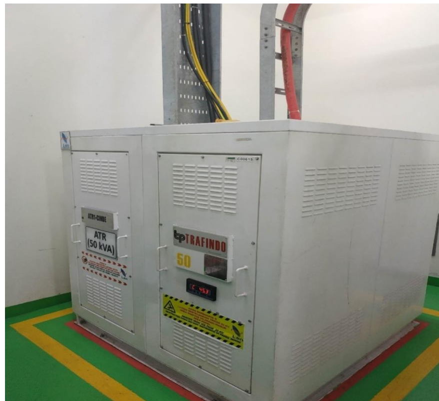
Gambar 2.21 Auxiliary Transformator
