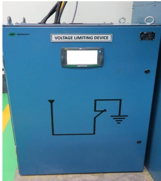
Gambar 2.18 Voltage Limiting Device Tampak Depan
